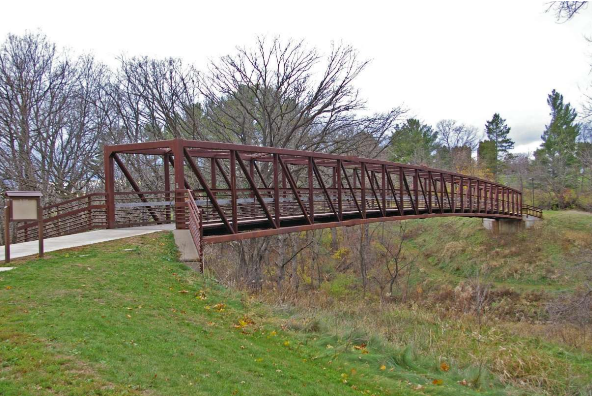
Figure 2: Pratt Truss
