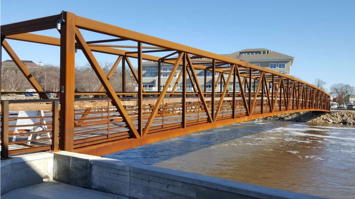
Figure 1: Warren Truss
